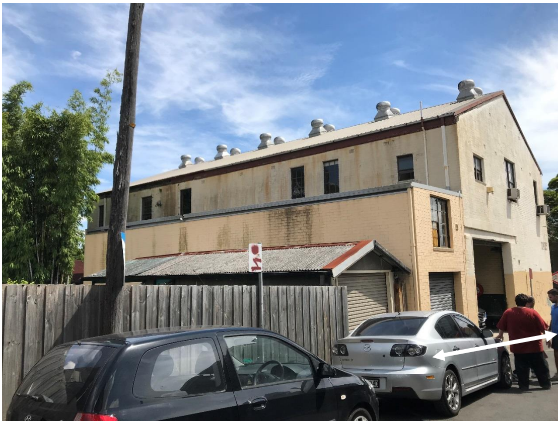
Figure 4: Rear elevation of existing building as viewed from Abels Lane.
