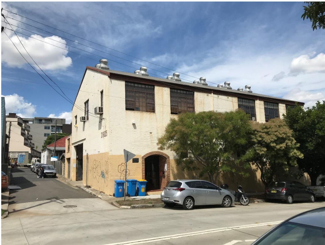
Figure 2: Site viewed from Trafalgar Street
