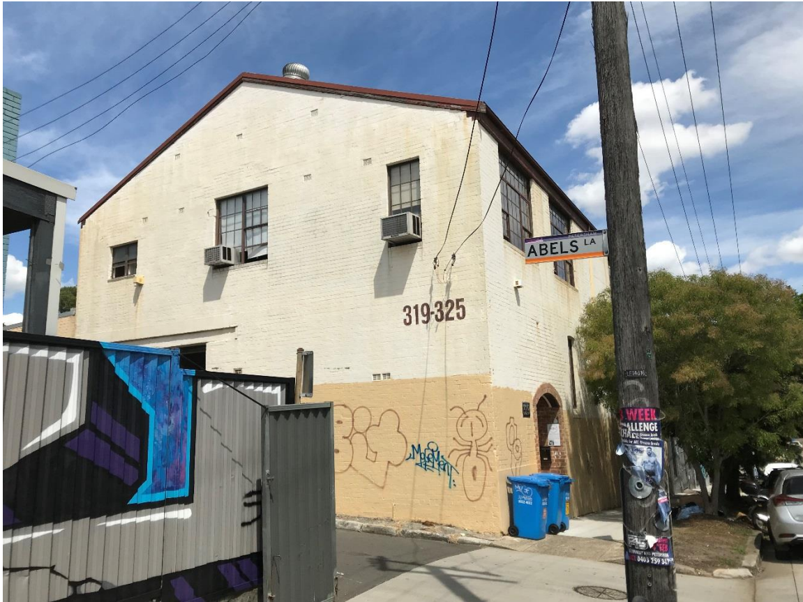
Figure 3: Eastern (side) elevation of existing building
